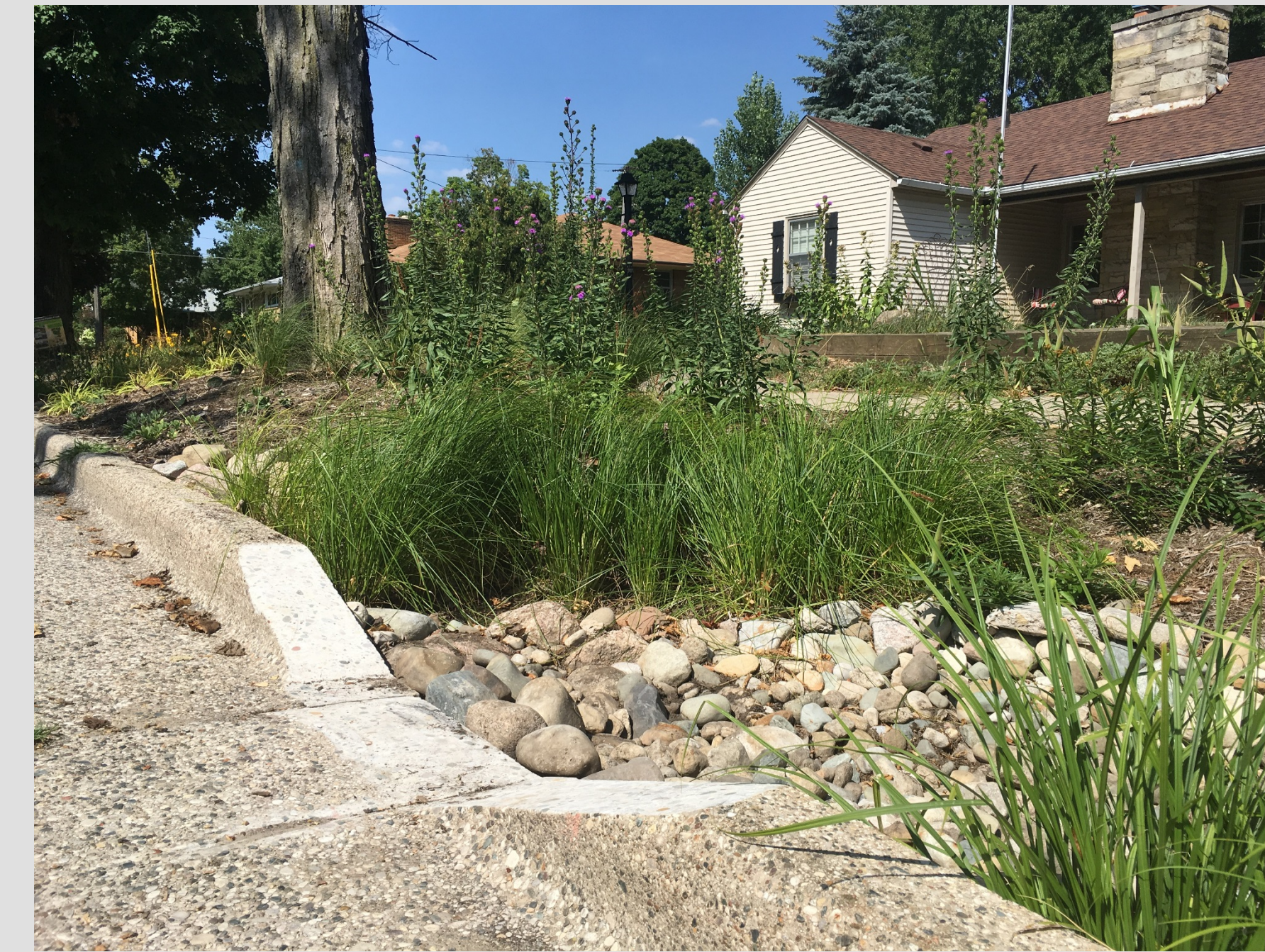
Figure- The cut curb of a mature rain garden in the Alger Heights neighborhood
